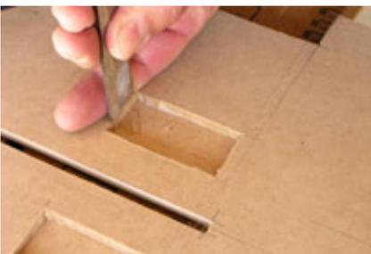
Step 3. Drill pilot holes for the doors and roof slots. It's a good idea to scribe the lines with a sharp knife before cutting with a jigsaw.
